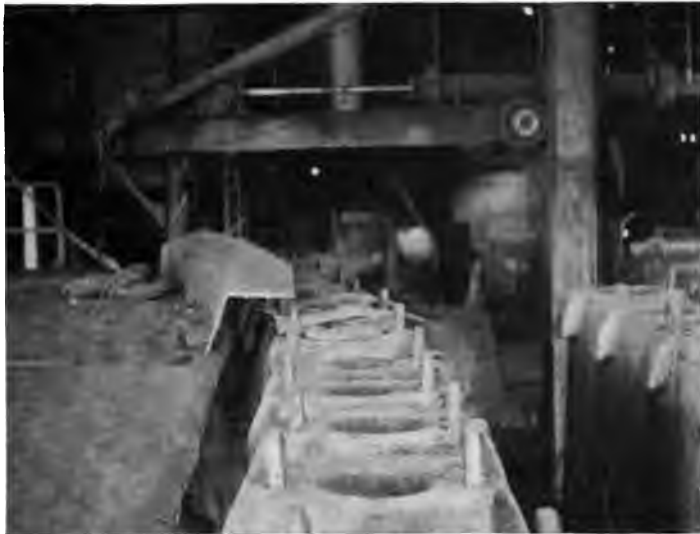
Fig. 1. Shield at the Edge of a Bessemer Pouring Platform.*
